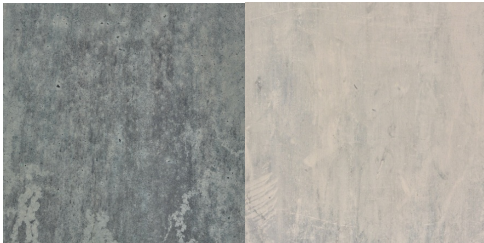
Figure 8. Example of images without defects.
